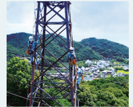
Construction of overhead electric power lines at a steel tower 100 meters above ground
