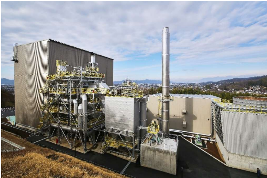
The Ashikaga Eco Power Plant
