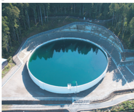
富山県南砺市 井波地区大型貯水槽 Large water tank in Inami district, Nanto City, Toyama
