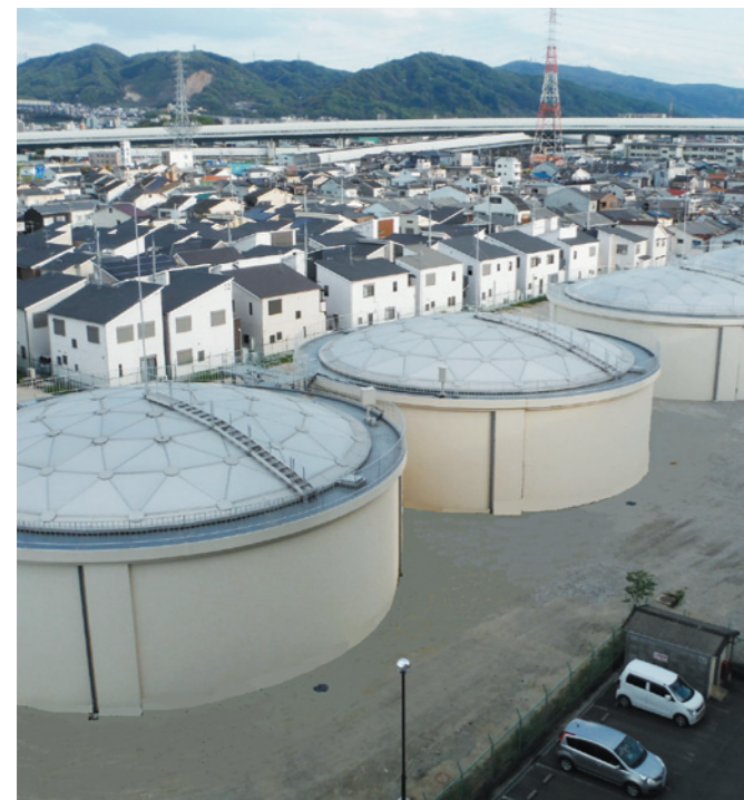
大阪府寝屋川市 楠根配水場受水池 Water distribution reservoir in Kusune, Neyagawa City, Osaka
