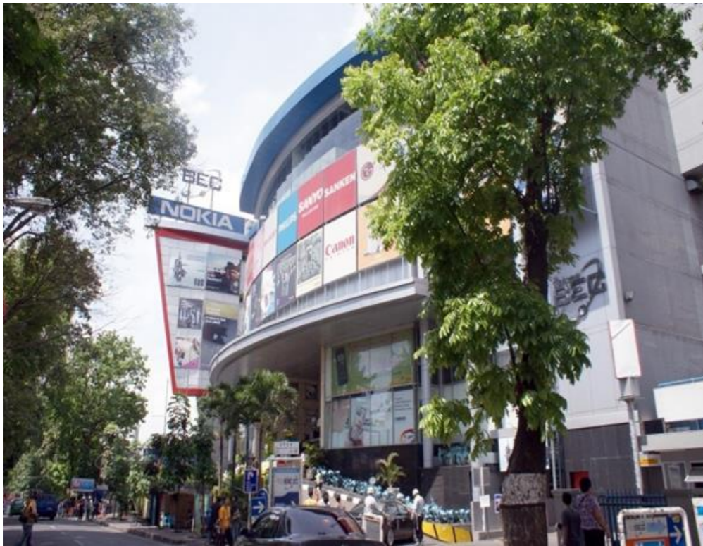
Shopping mall exterior
