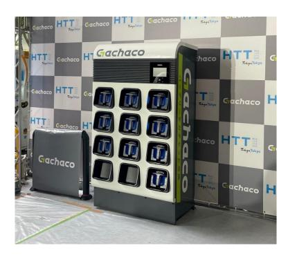
Battery exchange station for electric motorcycles, etc.
