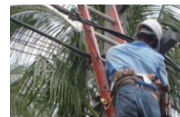
Optical access works (The Philippines) <MG EXEO NETWORK, INC.>
