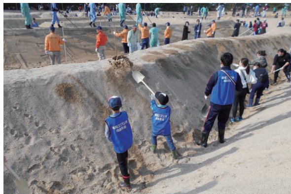
Sand arrangement using shovels
