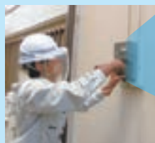
Installation of a smart meter
