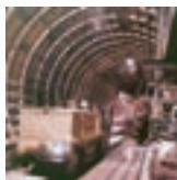
Engineering works adopting shield method
