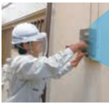
Installation of a smart meter
