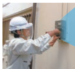
Installation of a smart meter
