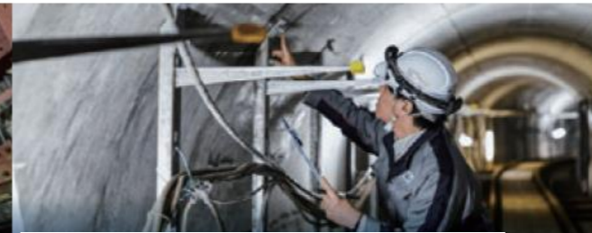
Maintenance work on underground facilities
