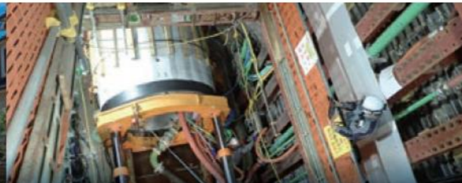
Tunnel construction with non-cutting method
