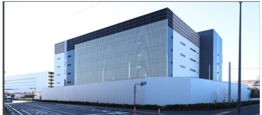
Building exterior photo
