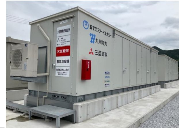
Grid Storage Batteries (NTT Anode Energy)
